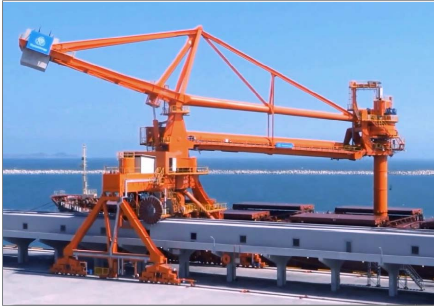
MCR on ship unloader for Zhuhai power plant ThyssenKrupp, China
